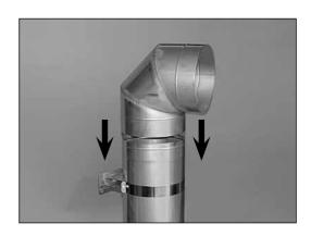
3. Align the pipe and elbow with the wall bracket and fasten it. 1 m distance must be between the finished floor and the middle of the elbow (see picture on page 3).
